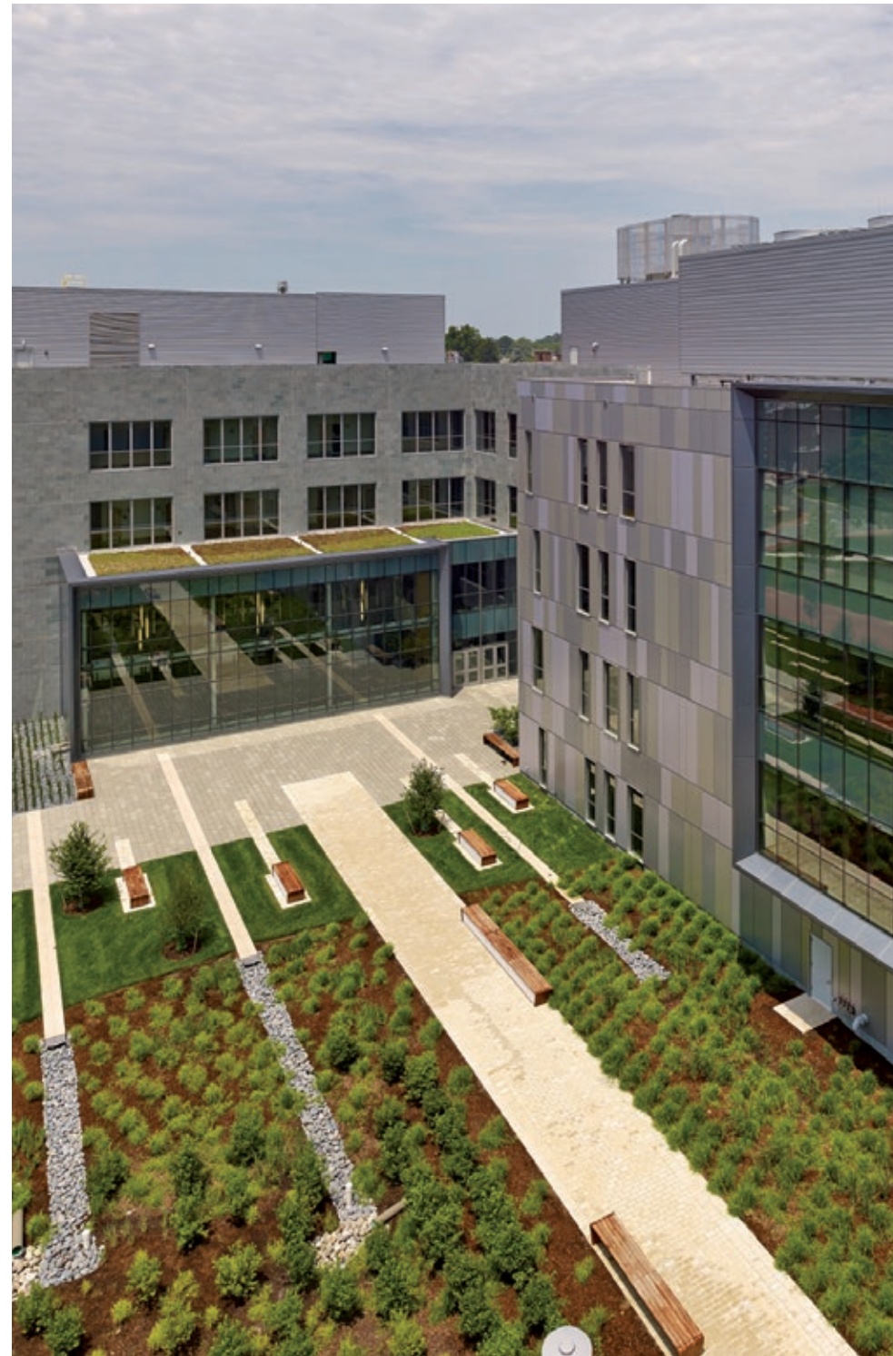
This project at the University of Delaware integrates stormwater management BMPs into aesthetic amenities that provide small gathering spaces to the university community.
