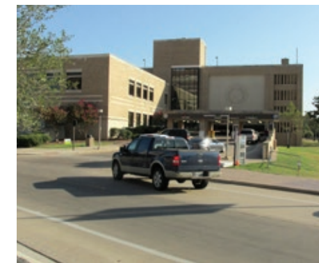
Parking structures provide good coverage for East Campus
