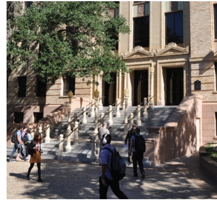
Entry at Chemistry (Note Non-Accessibility)
