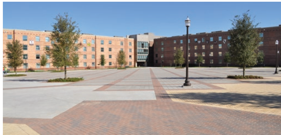
Renovation to Corps of Cadets Residence Halls and Quad
