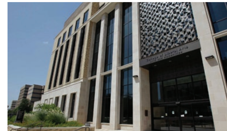
On-Building Signage at Liberal Arts and Humanities Building
