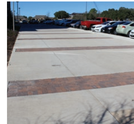
Fire Lane Paving
