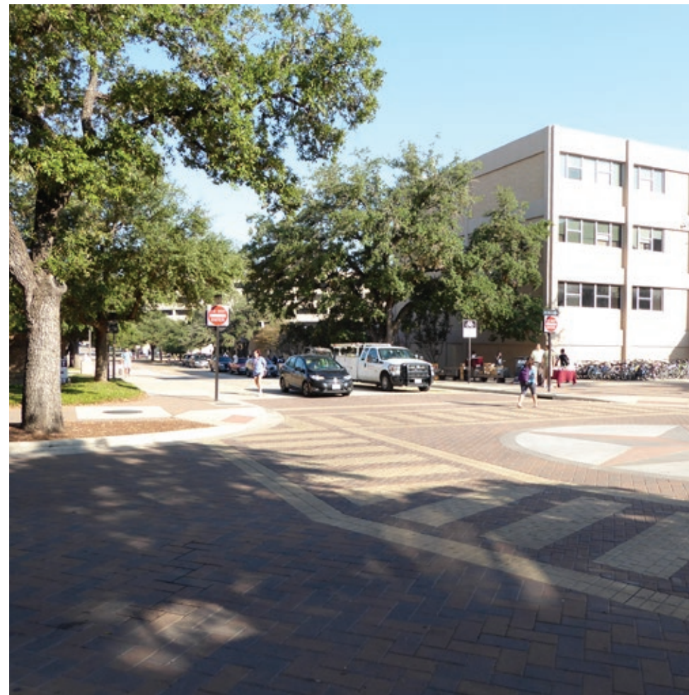
Paved Crosswalk in contrasting paver color
