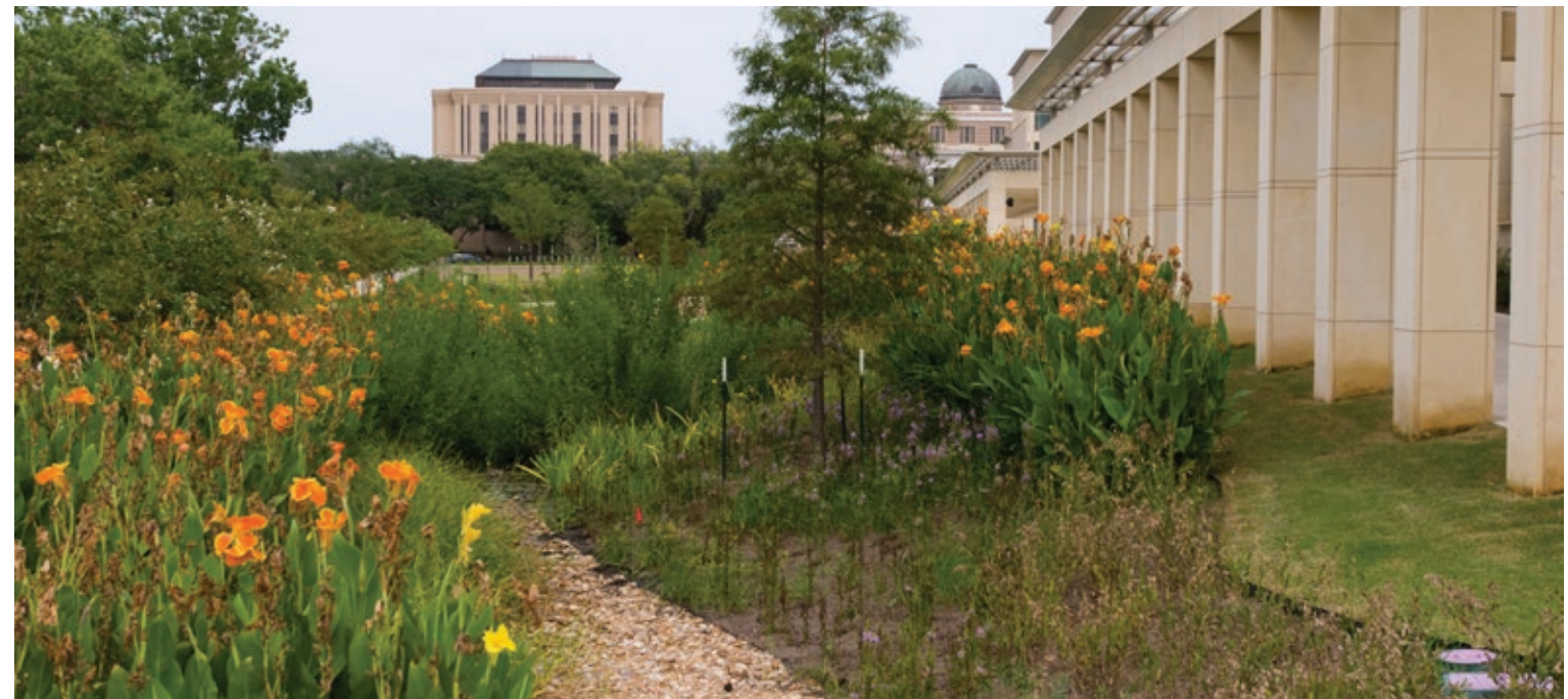
This rain garden at the Interdisciplinary Life Sciences Building manages stormwater while also providing a visual amenity and ecosystem services to campus.
