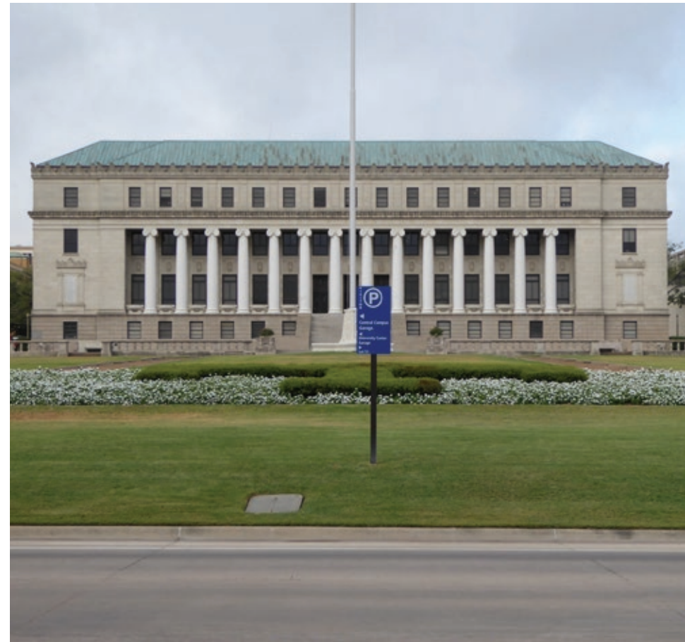
Visitor Parking sign placed in front of J.K. Williams Administration Building, which is an important vista for the campus.
