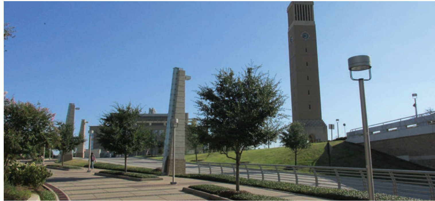
Underpass at Old Main Drive and Wellborn Road
