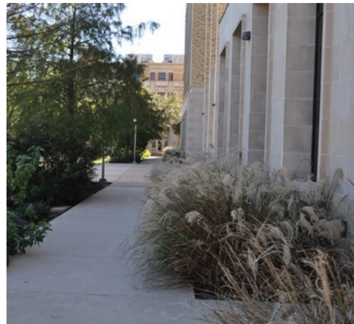
Limestone Masonry on Liberal Arts and Arts and Humanities Bldg.
