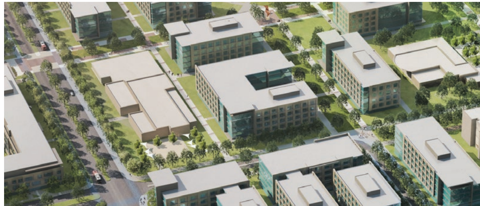
Pocket Park at SUP1 Addition - West Campus
