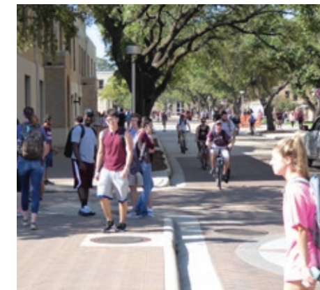
Concrete banding and curb
