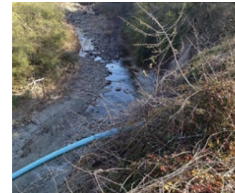
Erosion at White Creek
