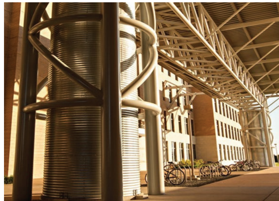
Rainwater Collection Cistern at Agriculture Building
