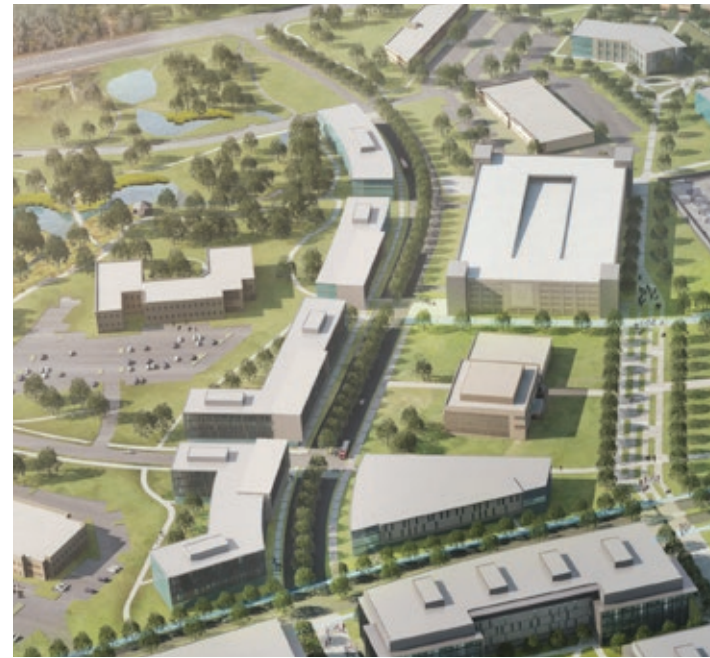
New Parking Garage on the Northwest of Research Park
