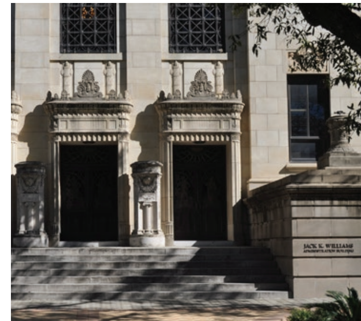
Limestone Masonry on Williams Administration Building
